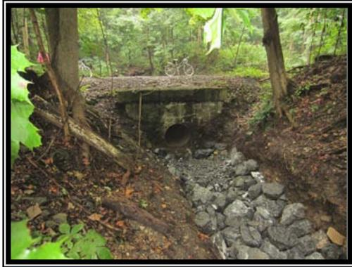
These culverts were totally clogged, collapsing and causing potential severe damage to the trail during heavy rains. Pepple's Excavating of New Enterprise repaired the culverts at a cost of just under \$24,000, funded through the same DCNR grant.
