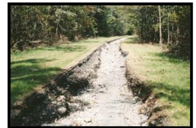
However, for those who weren't around at that time, the pictures show some of the damage to the trail caused by hurricane Ivan. As you can see in these pictures, the flooding caused by Ivan washed out significant portions of the trail from Williamsburg to Alfarata. The extent of the damage was horrendous. In some areas the gorge left after the waters receded was several feet deep.
